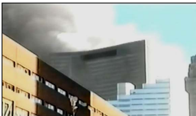
Classic Demolition Crimp in Rooftop of WTC-7
