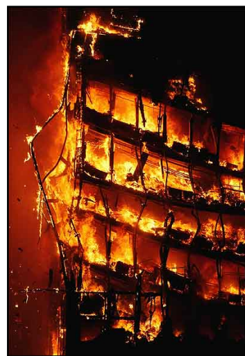
Windsor Building Fire Madrid Spain 2005
