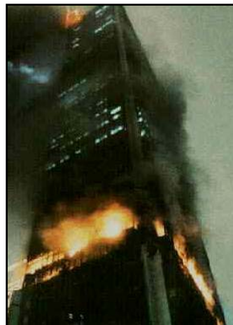
First Interstate Bank Fire Los Angeles 1988
