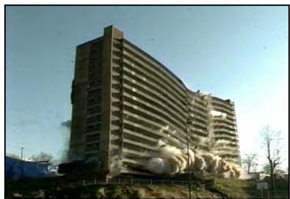
Classic Building Crimp from Demolitions
