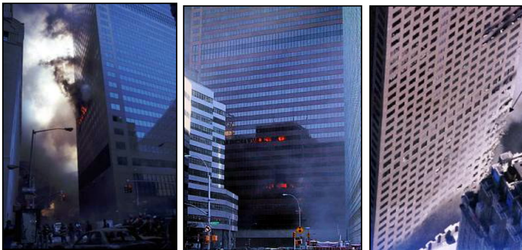
Minimal Fires of World Trade Center Building 7
