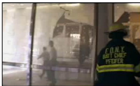
WTC Lobby Damage from Underground Blast
