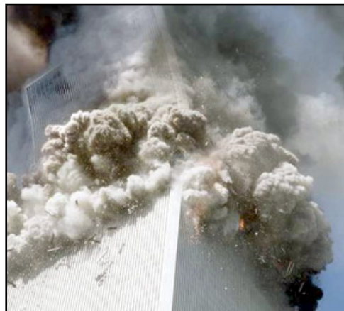
Top Floors Leaning Over the Center Axis 20°
